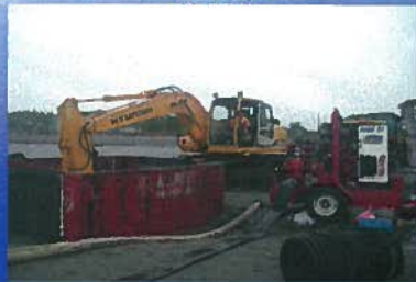
An excavator, shoring, and pumping were the main equipment used.
