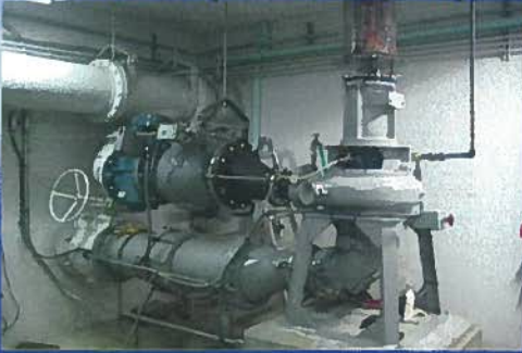
The completed 3 rd pump
