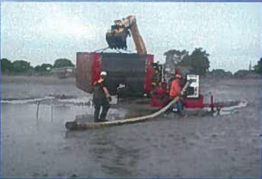
C. Johnson Construction started to setup.
