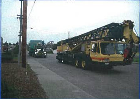
The Truck and Crane arrive on site.
