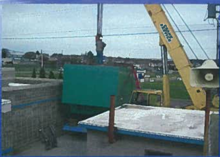
Hooking up for the lift.
