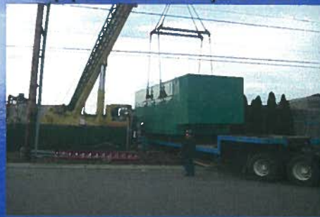
At nearly 40,000 pounds, it required large equipment and careful placement.
